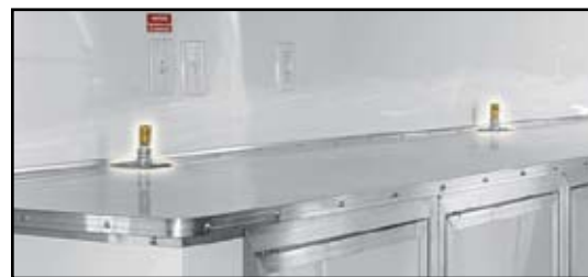
Air line connectors on a base cabinet with a stainless steel countertop
