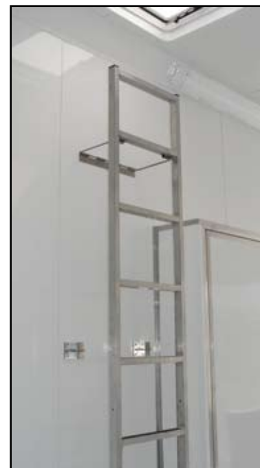
Folding ladder in open position. When not in use, ladder folds flat against wall.
